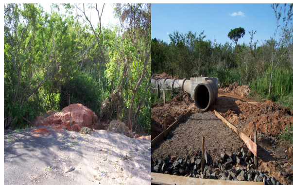
Figure 3 – Dirt street paved around the area and rainwater pipe built.
