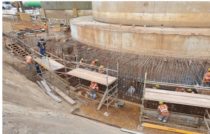
Figure 10 - Construction of the outer strengthening ring using the new piles executed.
