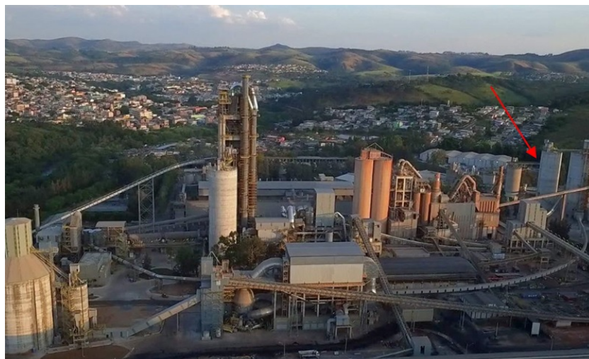
Figure 12 - Detail of the position of the strengthened silo within the industrial complex.
