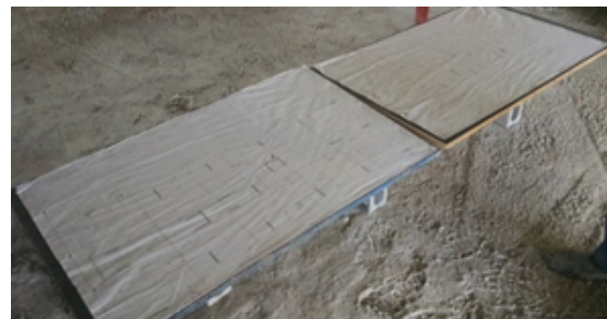
Figure 5 – Marking project laid out on the pavement.
