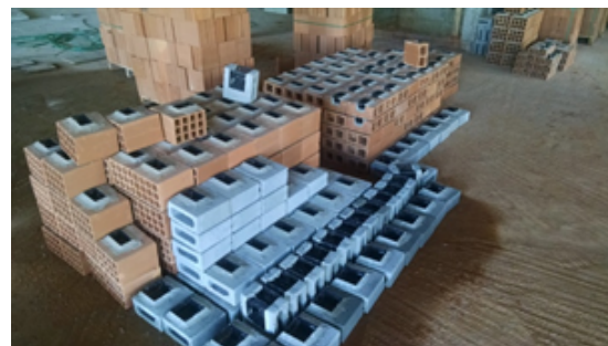
Figure 7 – Block stock beside the anchoring center.
