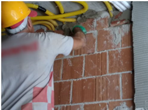
Figure 11 – Execution of wedging.
