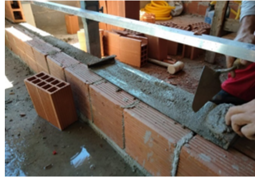
Figure 6 – Laying mortar after using the gutter.
