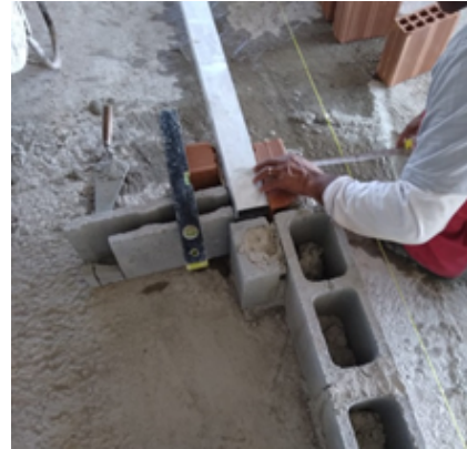
Figure 4 – Laying the first block of the course.
