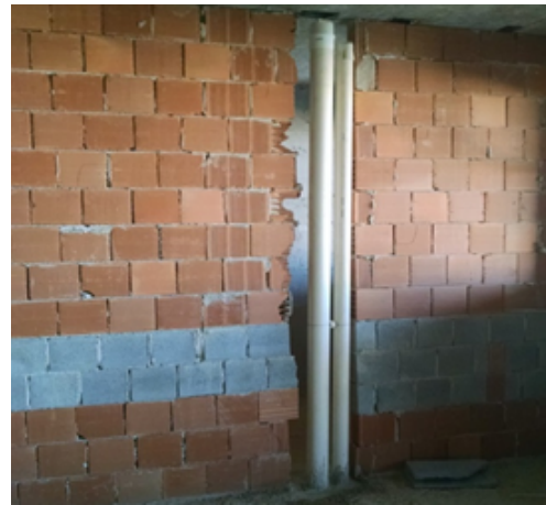
Figure 9 – Segmentation of the wall for passage of the plumb line.
